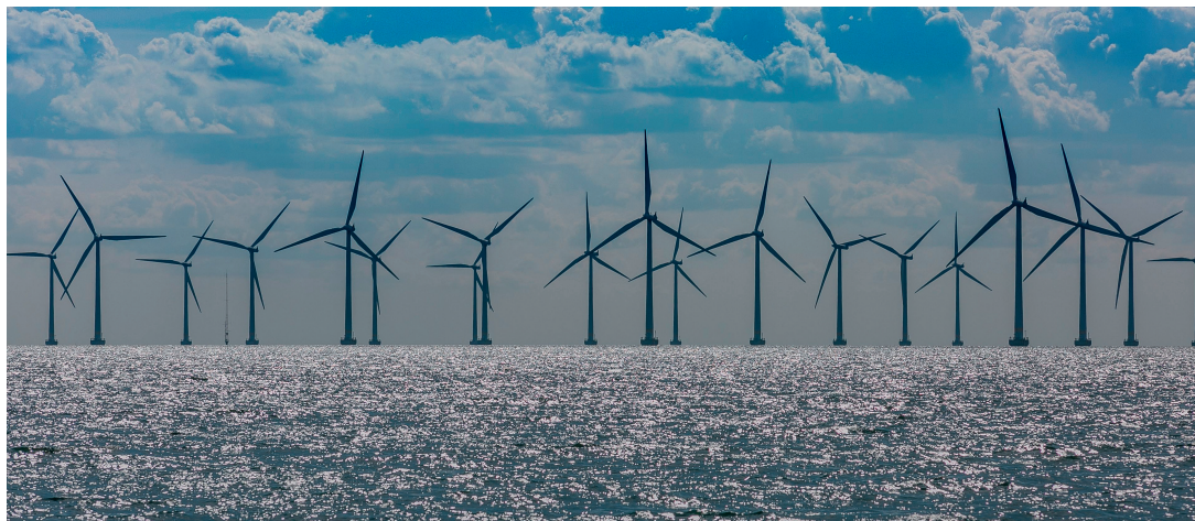
Fig. 4. Leading edge erosion is a challenge for large commercial wind turbine blades. Protection against this is provided by a so-called Armour-Edge shield made from the styrene copolymer Luran SC.
